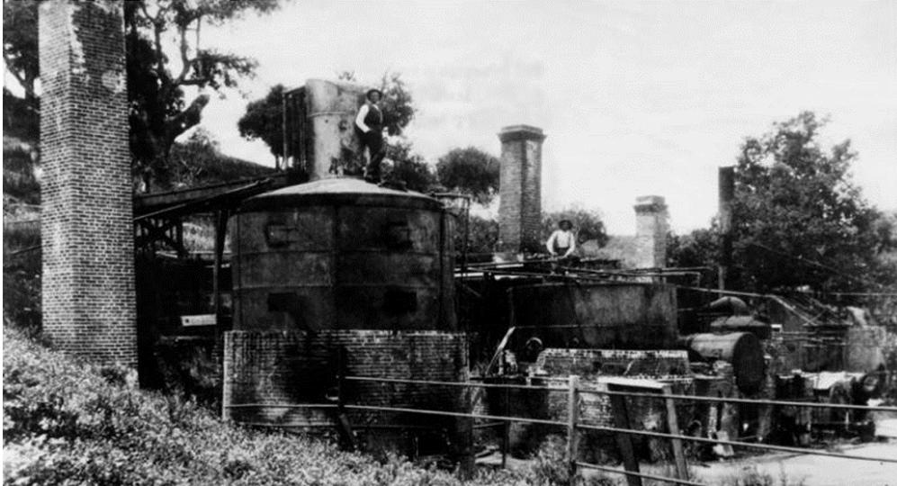
**Figure 2** All four Stills (left), intact condenser to the rear of Stills, and Residuum Tank (right), date unknown; Security Pacific National Bank Collection, Los Angeles Public Library
